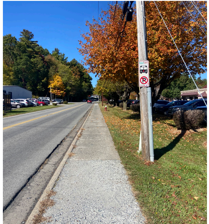
Existing utilities along back of existing sidewalk on Greenway Road
